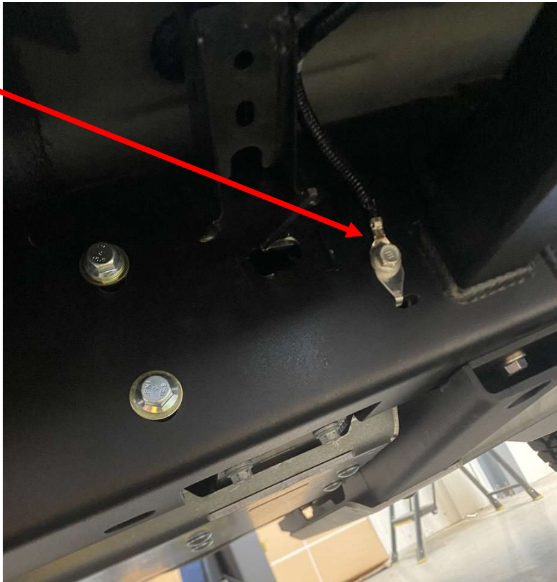
Figure 7: Ground wire reinstalled correctly.
