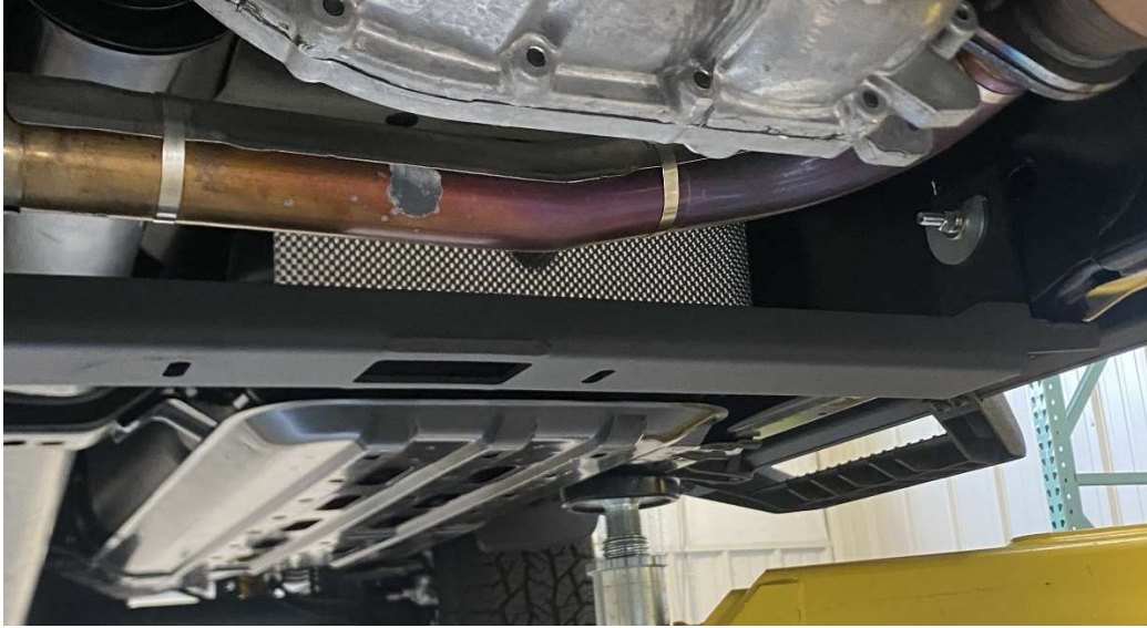
Figure 4: Correctly installed crossmember.
