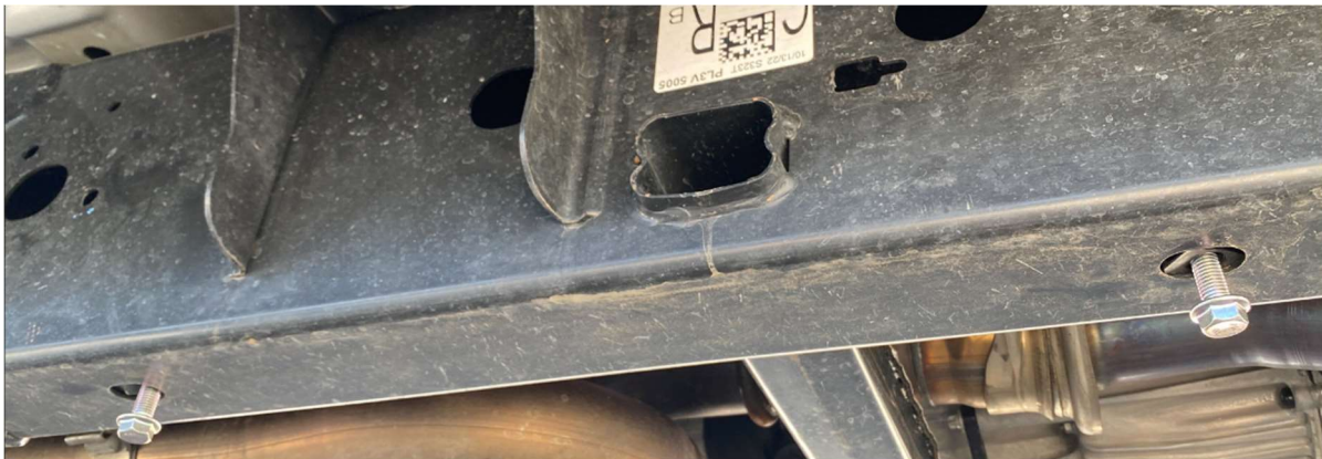
Figure 16: Preinstallation of Lower M10 Bolt
