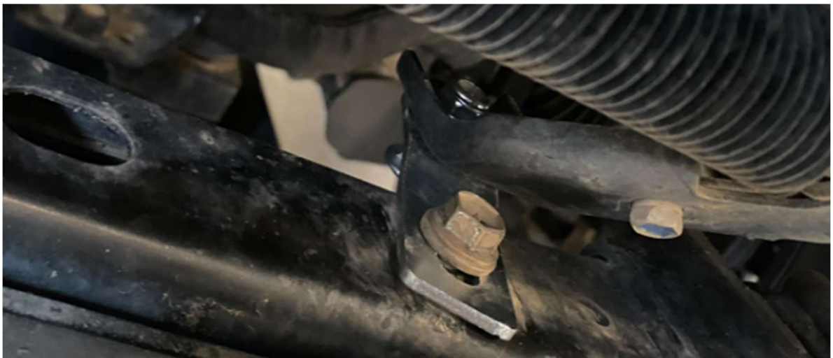
Figure 13: Correct installation of frontmost brackets.
