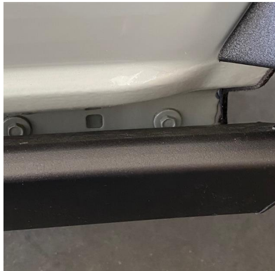
Figure 3: Frontmost pinch weld bolts
