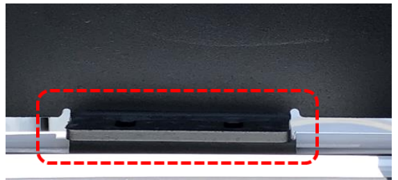
Figure 10: Rubber mounting block
